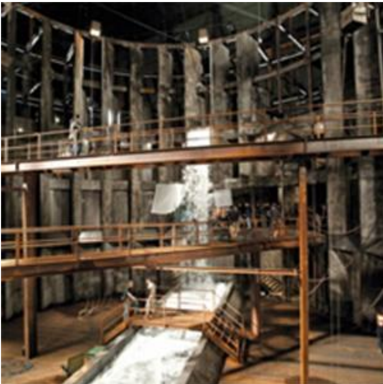
Figure 2 – more detailed view of the sewer
